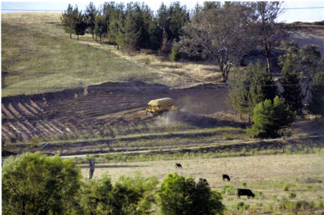
New quarry access road under construction 11 Dec 2013 6.40 pm
