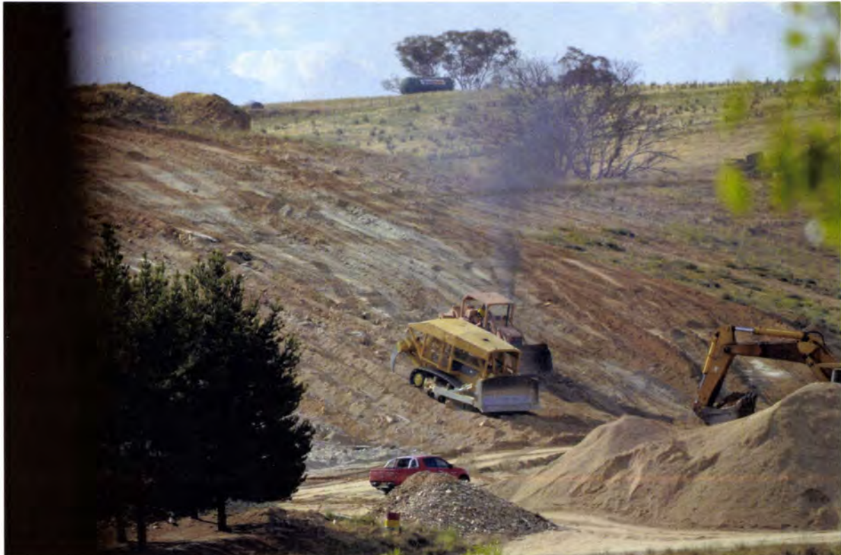
Two bulldozers and excavator extract gravel 17 Dec 2013 5.25pm
