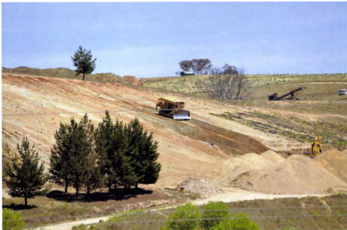
Excavations in progress Sunday afternoon, 1 December 2013. Noise from this gravel extraction process is the loudest and most intrusive.
