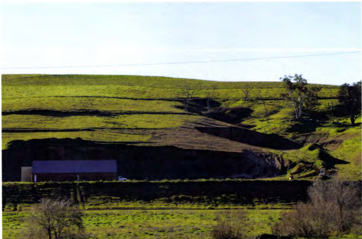
Excavated gully pictured on right falls outside proposed quarry area with no plan for rehabilitation
