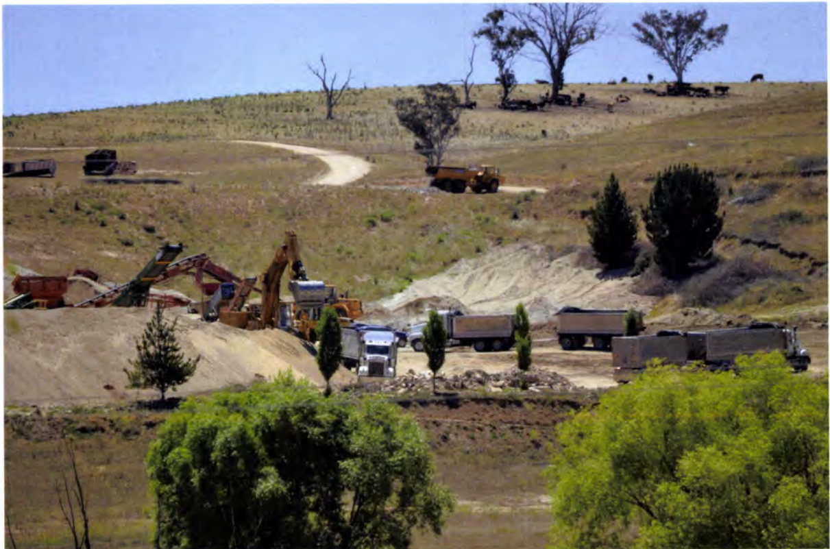
13 Dec 2013. Three trucks of many which cycled throughout quarry hourly from 6.30 am to 4pm
