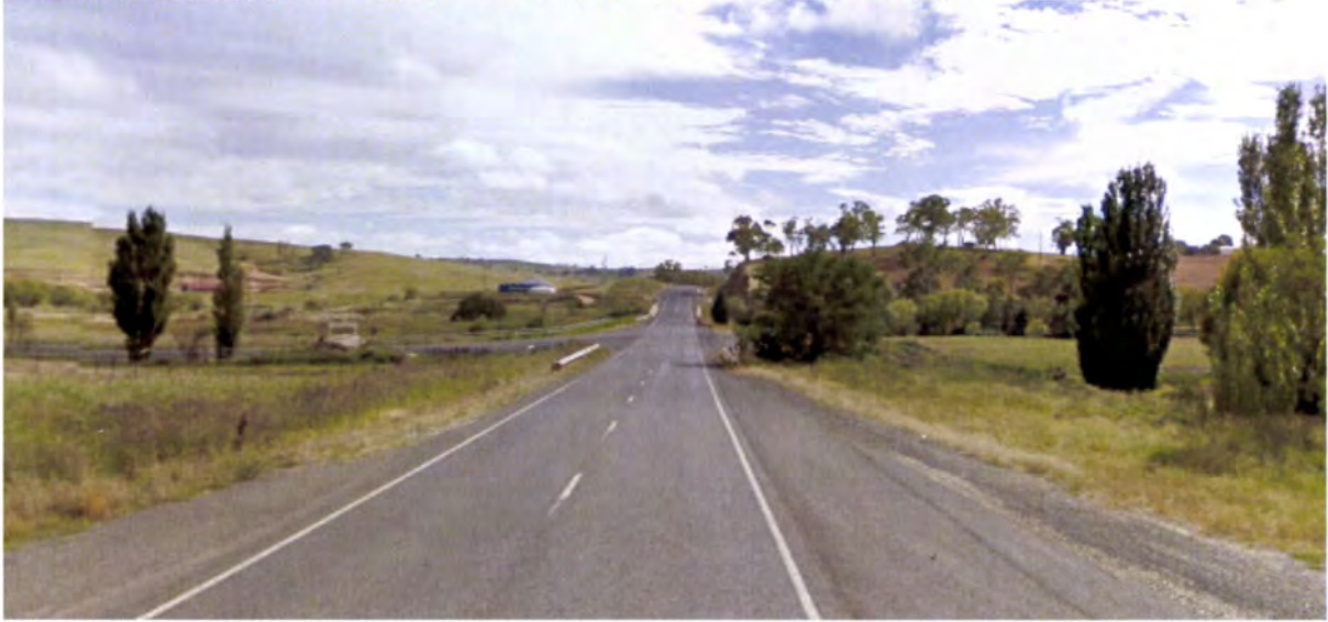
Photo 3: Existing access to the subject land viewed from the south
